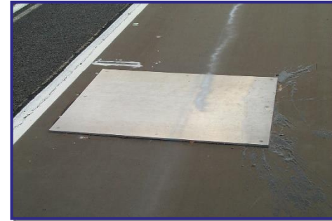
Plate on the track
