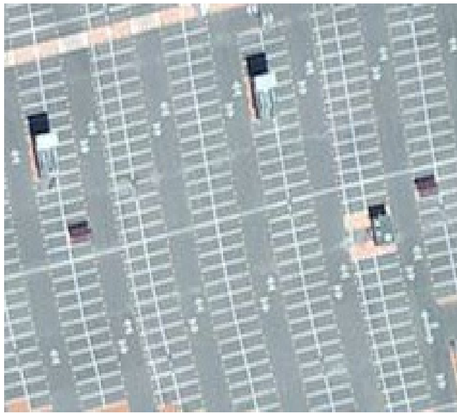
(a) A car park? No, the roof of a small used as a car park.
